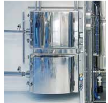
Filter housing for Bag-In-Bag-Out changing of HEPA filter element.
